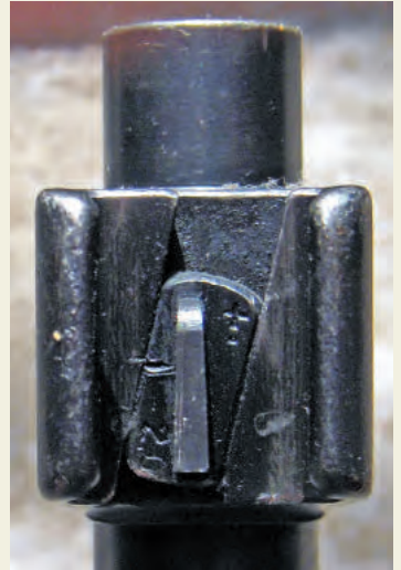
Top view of K31 front sight residing in its angled dovetail.
